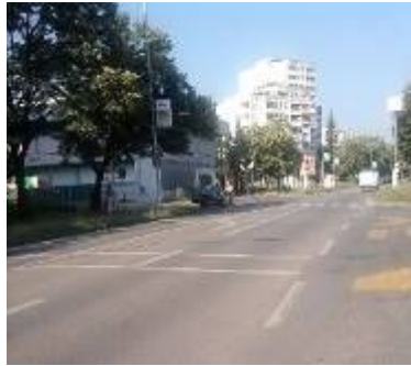
Vibration strips in Borik
