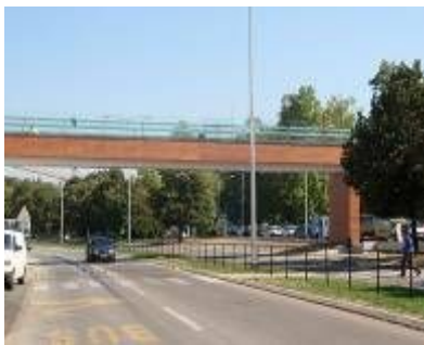
Over road footbridge
