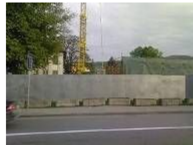
Protective fence on the construction area
